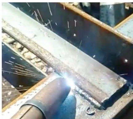
MIG Welding Process
