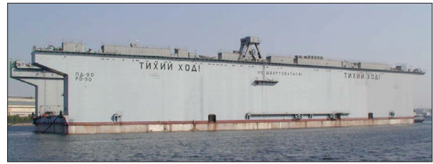
Fig. 6. Repair composite floating dock with the buoyant power of 13,500 tones before delivery to the Russian Federation
