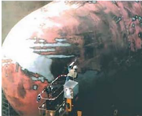
Figure 14.2 – The old paint-layer is removed by gritblasting [21]
