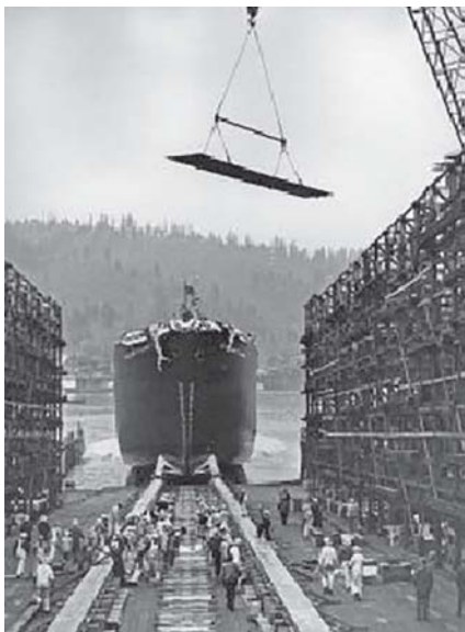
Figure 13.8 – Longitudinal oiled slideway launching [1]
